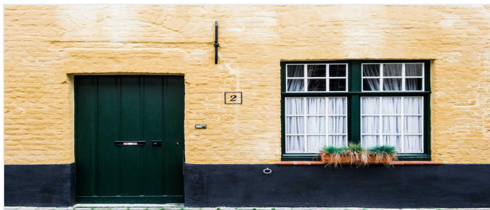
Banner monteret - frontfacade
